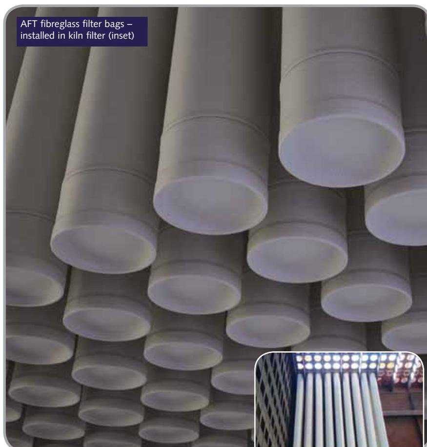
AFT fibreglass filter bags – installed in kiln filter (inset)
