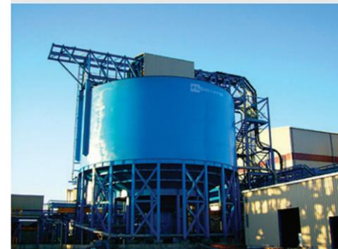
EIMCO Deep Cone paste thickeners produce underflows concentrated to near their limit of pumpability. The deep tank design maximises solids concentration, and produces uniform, non-segregating underflow slurry with a paste consistency.
