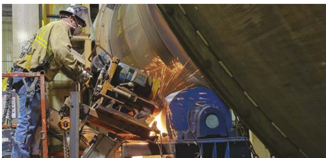
Support roller grinding
