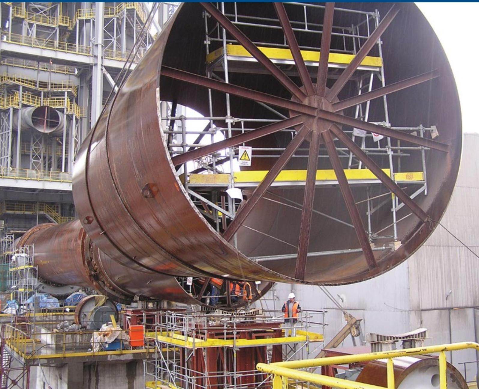
**FLSmidth provides expertise to supply, install, maintain and repair kilns on-site at plants around the world, irrespective of the OEM.**
