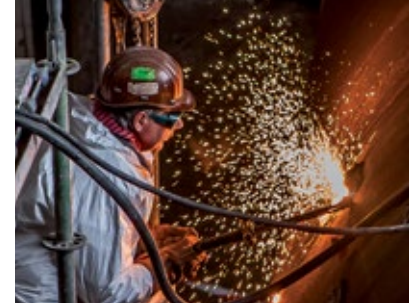
Cutting of kiln shell
