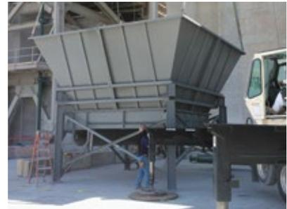
*Volumetric unit for AF utilization during installation*
