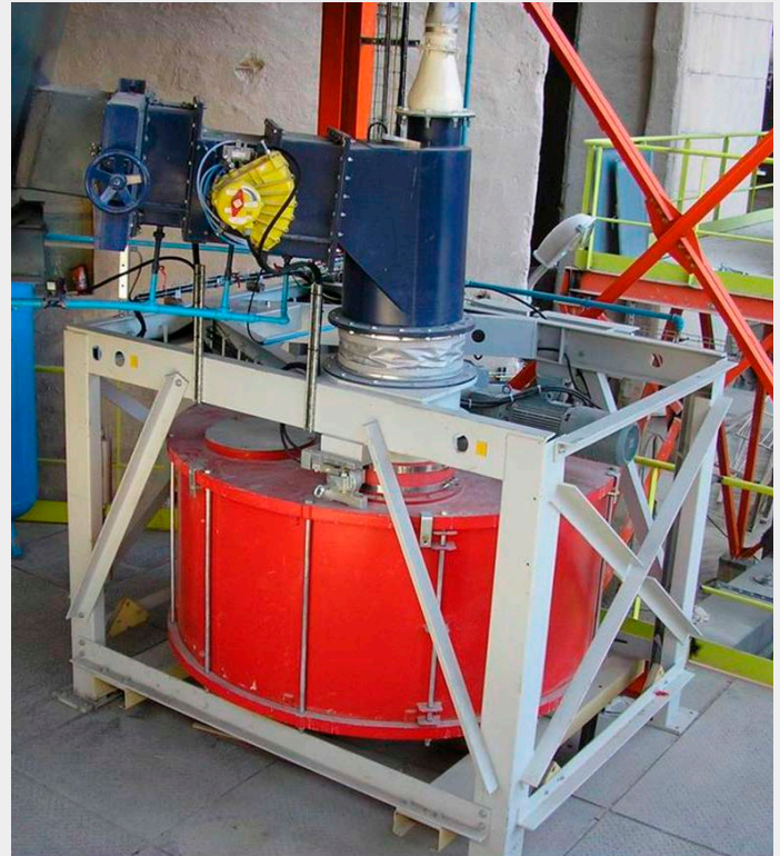
Kiln feed installation at a clinker production line in Romania.
