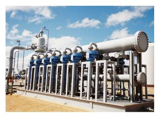
Each engineered system is designed to meet or exceed applicable standards. We offer almost any material of construction, including carbon steel and exotic alloys. Hydrocyclone liner material is wear resistant alumina ceramic or silicon carbide lining, depending on the application.
