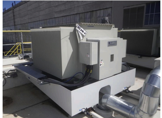
Fig. 6. Close view of one of the MPPSs after installation.
