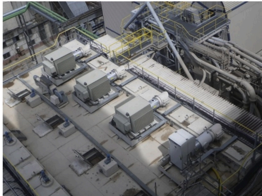
Fig. 5. Aerial view of the roof of the ESP.
