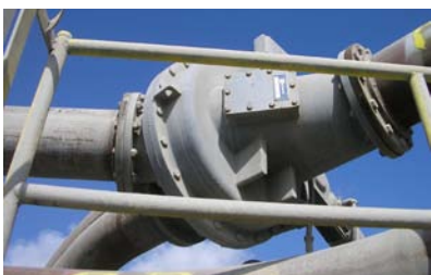
2-way SK diverter valve
