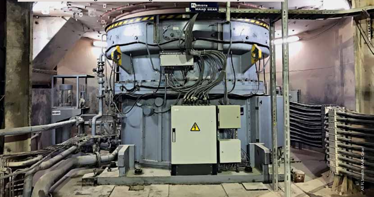
The FLSmidth MAAG Gear CEM Drive
